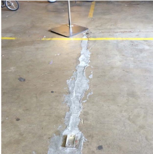
Photo #5: Repairs to cracks in concrete on main shop floor
