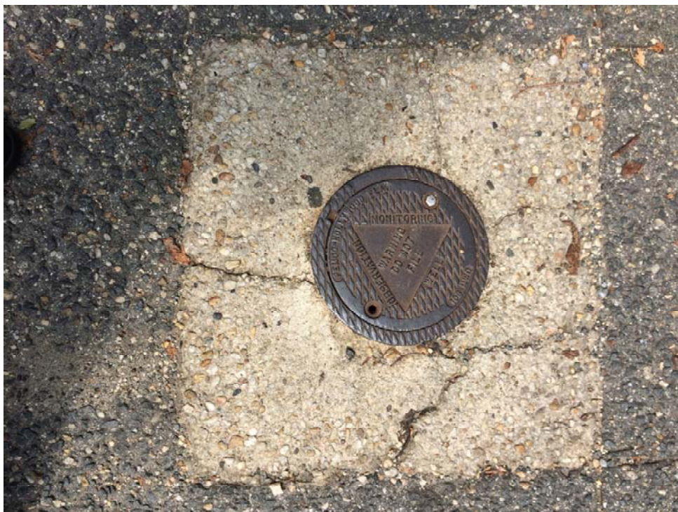
Photo #2: Existing monitoring well located in yard to the north of the building
