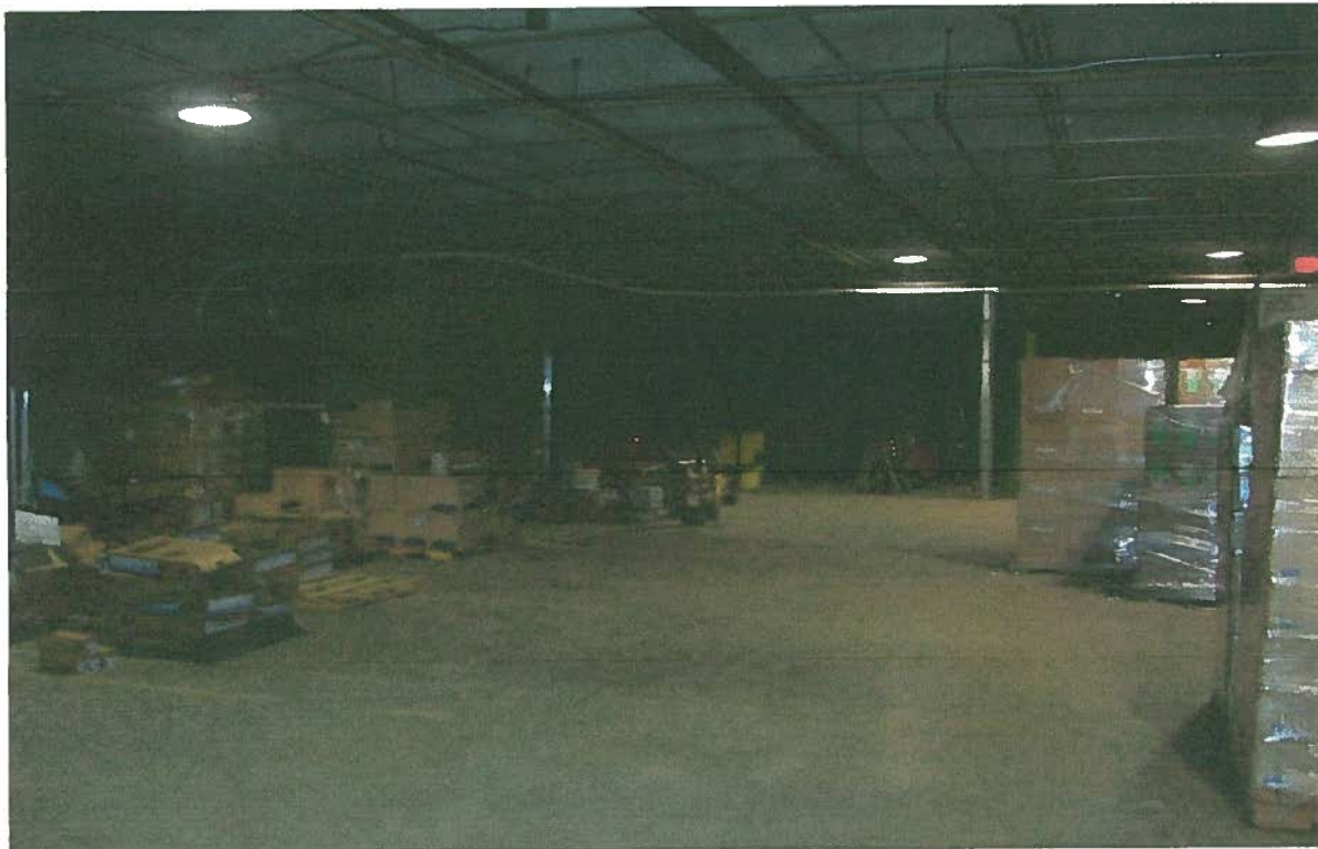
Internal View of Subject Property
