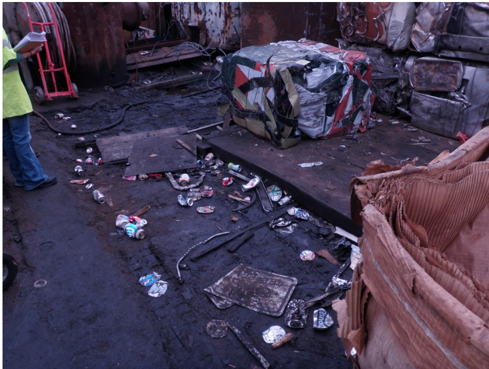
Photo #4: Staining of concrete in Square 0605, Lot 0802
