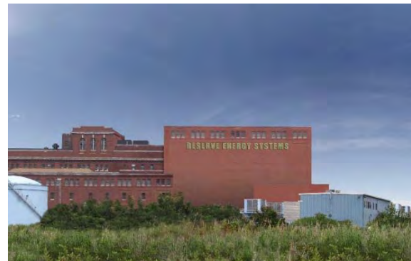
CSWS Power Block Facility – After
