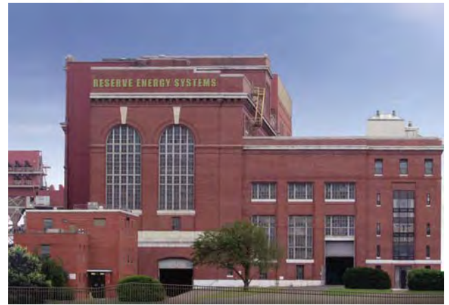
CSWS Power Block Facility, Hartford - Redeveloped
