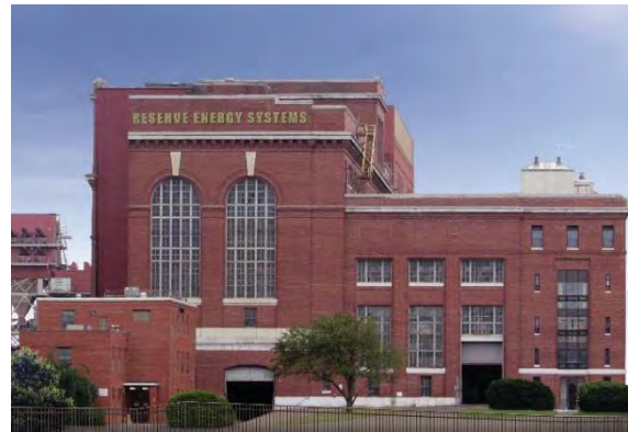
CSWS Power Block Facility – After
